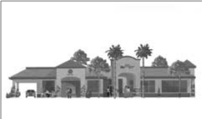
Yuba City Opened April 15, 2002 1600 Butte House Road • Yuba City, CA 95993 (530) 751-2700
